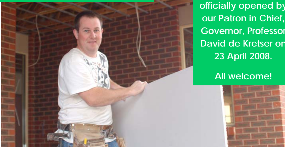
Luke Flower works on the plastering at the new facility.
